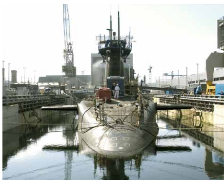
Devonport Royal Dockyard, United Kingdom Courtesy of Devonport Royal Dockyard Limited
